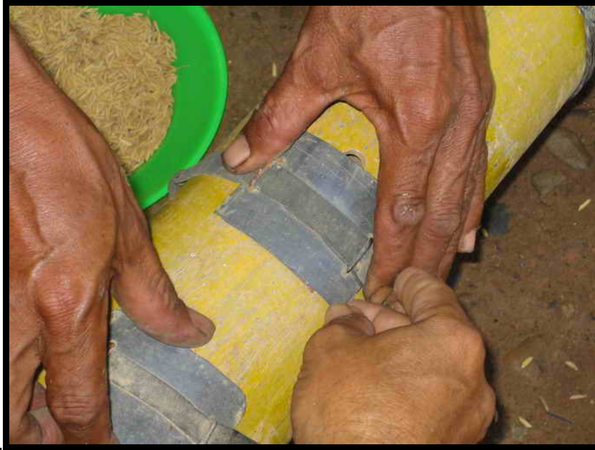
Figure 3. Close the Hole with Rubber Belt.
